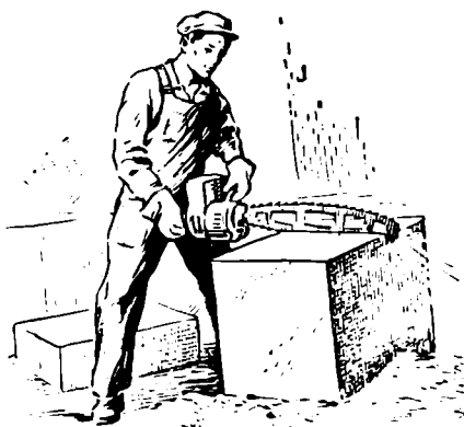
Fig. 310. Sawing a coquina block with a power saw
